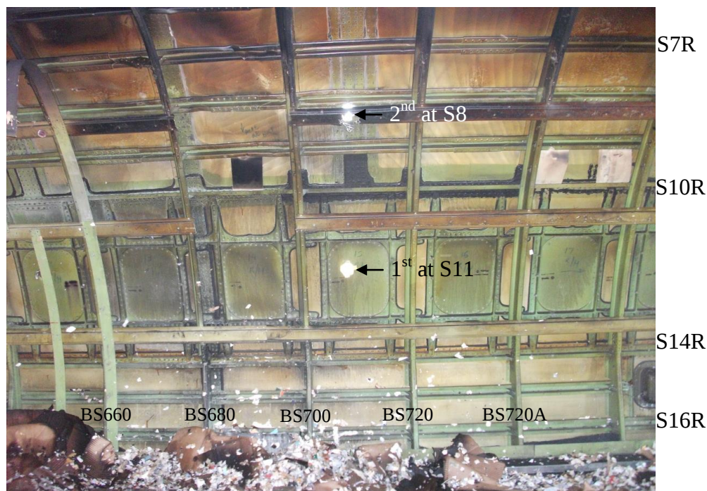
Figure 20. Interior view of lower STBD side.
