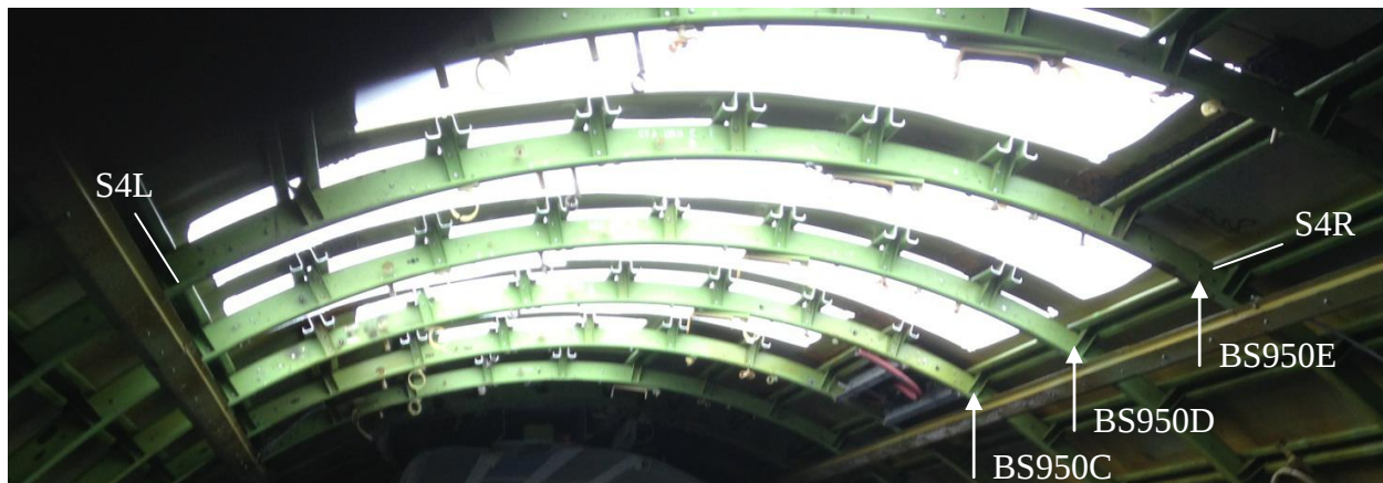
Figure 11: Skin sections and stringers removed.
