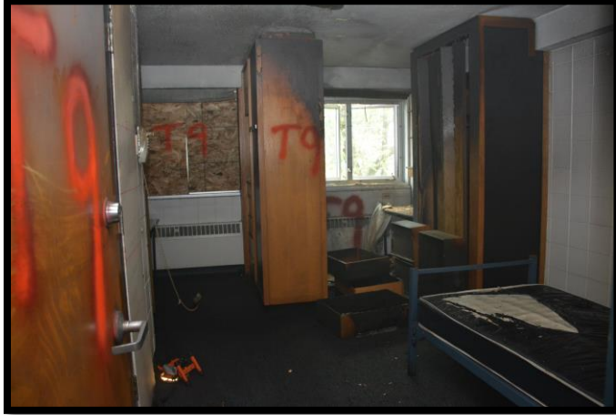
Figure 43-T9 UHP 19.6 second flow 9.8 gallons
