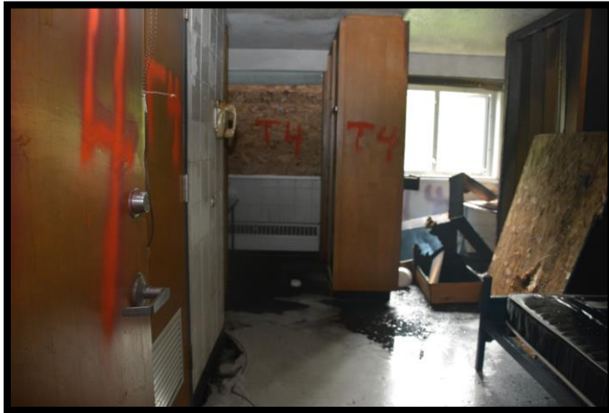
Figure 38-T4 Fog Nozzle 6.22 second flow 15.5 gallons
