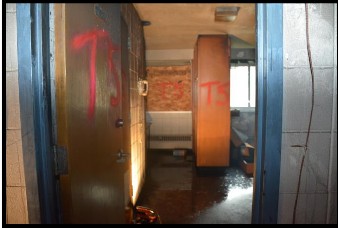
Figure 39-T5 Fog Nozzle 16.4 second flow 41 gallons
