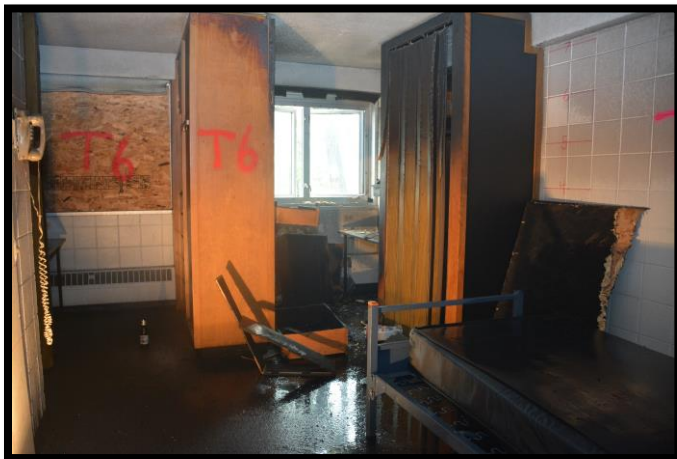
Figure 40-T6 Fog Nozzle 10.27 second flow 25.7 gallons
