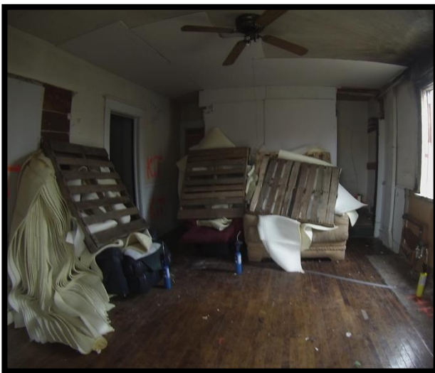
Figure 24-T14/T15 Fuel Load A/D First Floor Room
